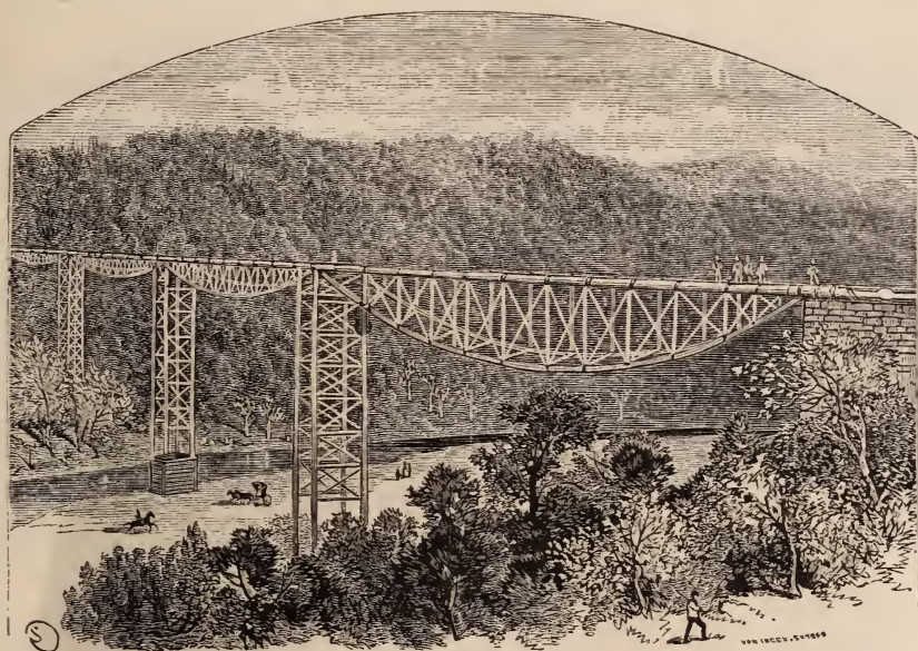
THE PIPE BRIDGE OVER THE WISSAHICKON.
